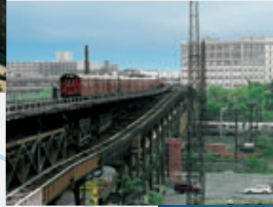
Sunnyside Intermodal Facility, Planning Queens, New York Ehrenkrantz Eckstut & Kuhn Architects/WAI JV
